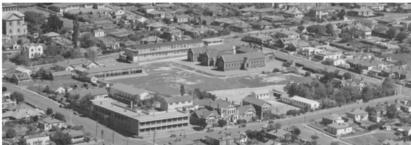
An aerial photo of the old and new school buildings in 1956 with the Technical College in the foreground. The infant block at left of the Main School site opened in 1940.
